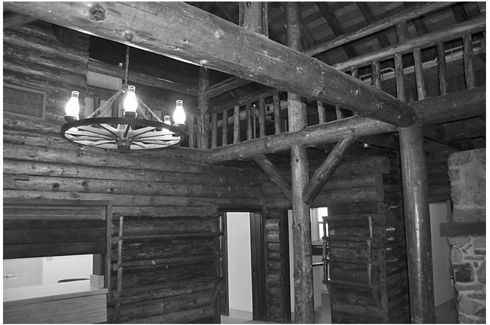
Structure of the lodge's main room and balcony Riverside Co. Parks
