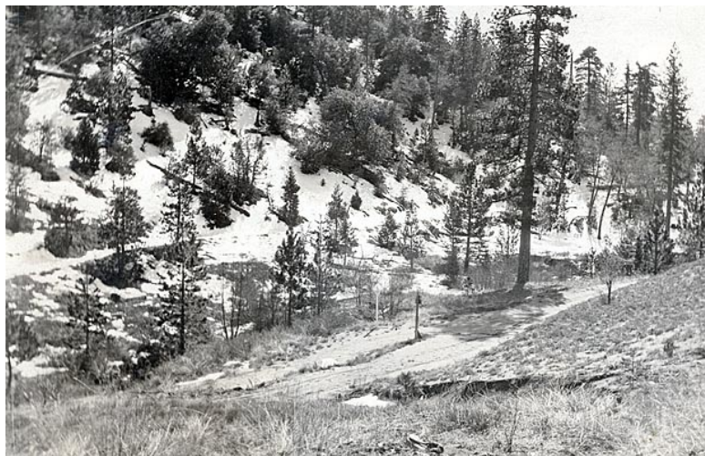
The 1910 road's detour up Hall Canyon is still visible above the shores on both sides of Lake Fulmor. —IAH archive
